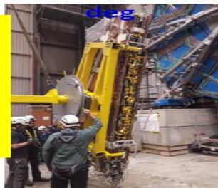
Set orientation to 22.5 deg Installation Fixation on NSW A
