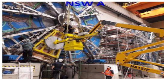
Set orientation to 22.5 deg Installation Fixation on NSW A
