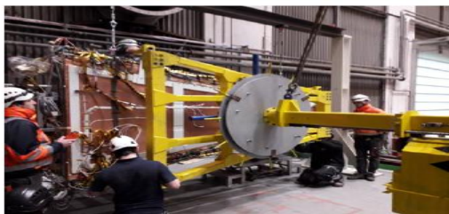
Set orientation to 22.5 deg Installation Fixation on NSW A
